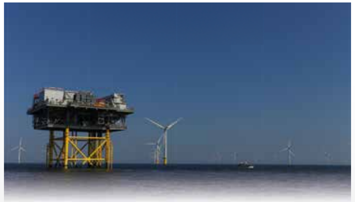
Off-shore platforms WORLDWIDE
