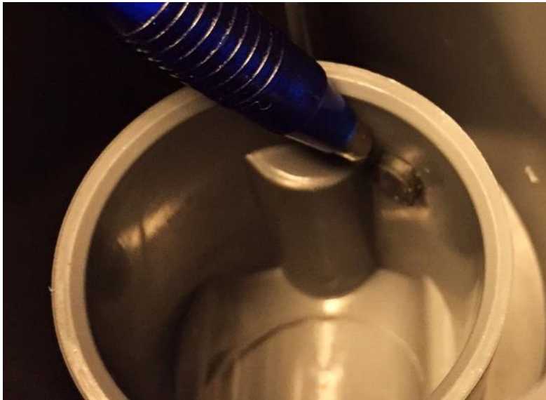
Figure 72: Pressure side installation: remove the black closing plug
