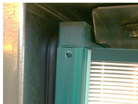
Figure 53: Check, if filter lie on the sealing
