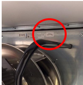
Figure 74: Rotation marking of EC fans
