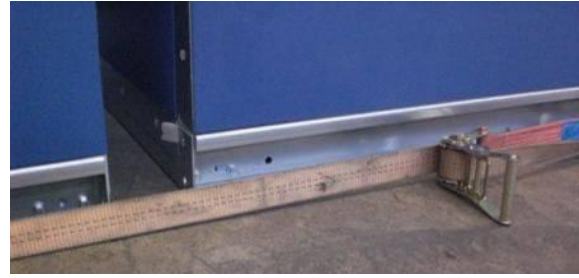
Figure 24: Pulling AHU sections together (detail)
