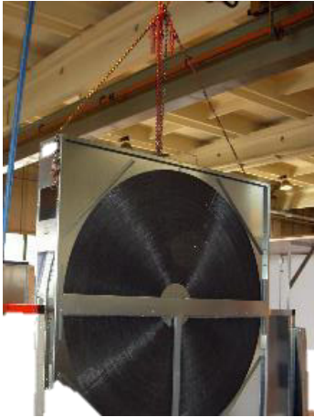
Figure 85: Lifting with chain hoist
