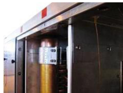
Figure 61: Mounted STRAUB coupling
