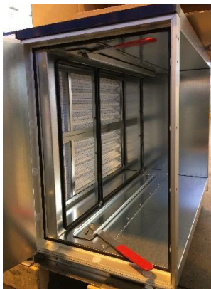
Figure 49: Filter frame for different filter sizes
