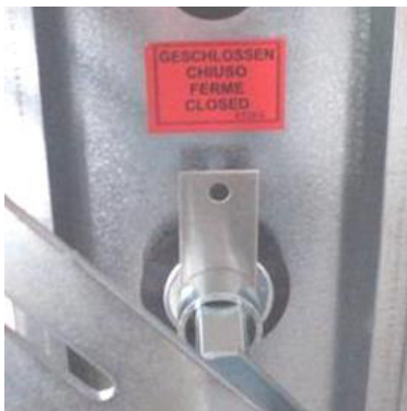
Figure 43: Closed position, characterized by a sheet metal position indicator
