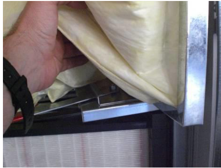
Figure 48: Lifting the filter bags
