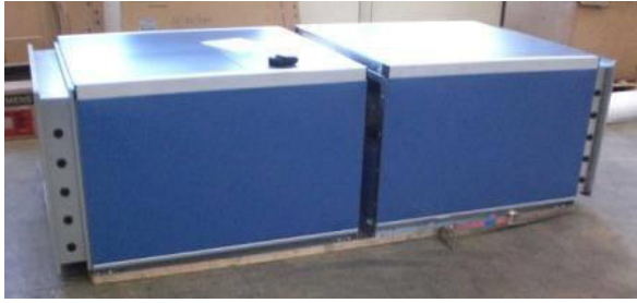
Figure 23: Pulling AHU sections together
