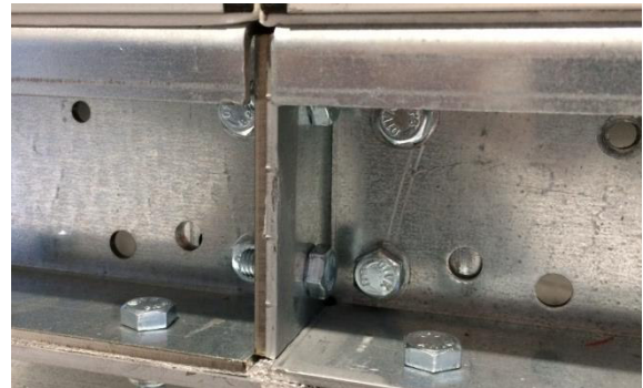
Figure 26: Bolt connection of base frames
