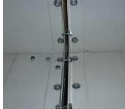
Figure 31: Connection via connection strengthening angle
