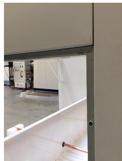
Figure 139: Door frame without door panel (TRA-E)
