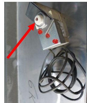
Figure 212: Thermostat with uncovered reset button
