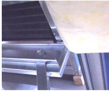
Figure 153: Slide in the filters
