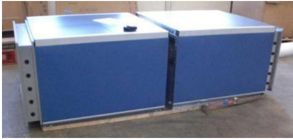
Figure 56: Pulling AHU sections together
