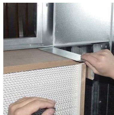
Figure 162: Inserting the filter cell
