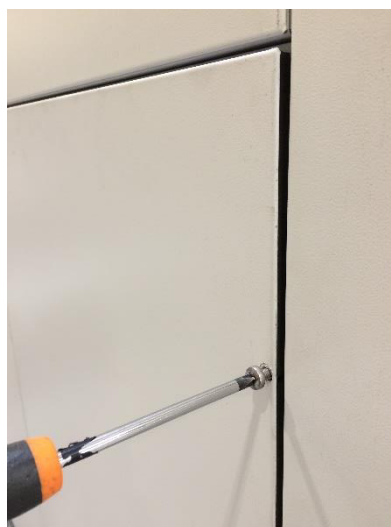
Figure 138: Undoing the screw and removing the door panel (TRA-E) from the door frame
