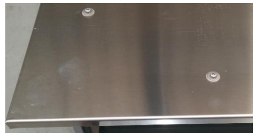
Figure 110: Metal sheet roof mounted
