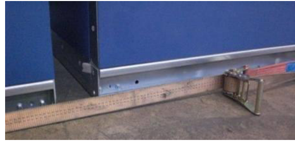
Figure 57: Pulling AHU sections together (detail)
