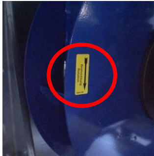
Figure 206: Rotation marking of plug fans
