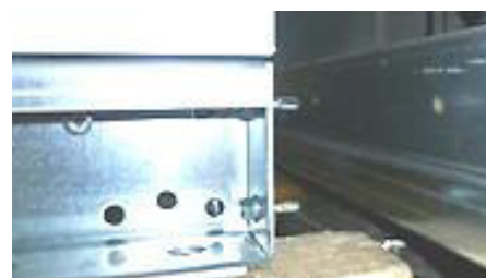
Figure 80: Application of self-tapping screws
