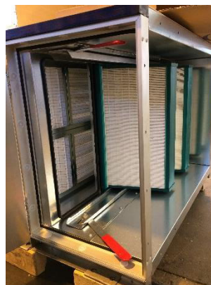
Figure 157: Consider the order according to the filter frame raster
