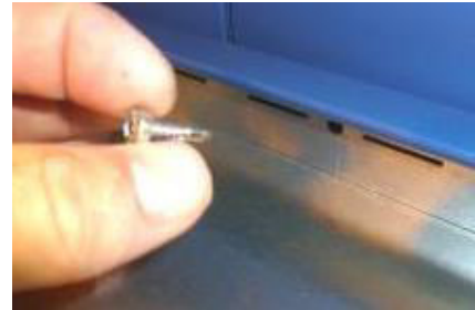
Figure 83: Joint at the AHU
