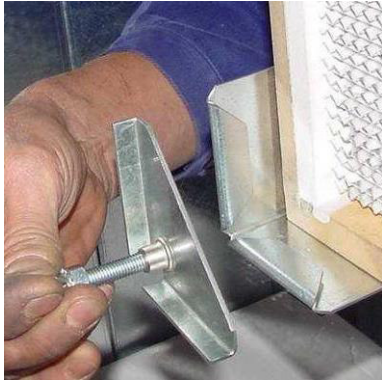
Figure 163: Inserting the clamps
