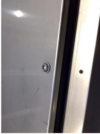
Figure 60: Fitting the external panels
