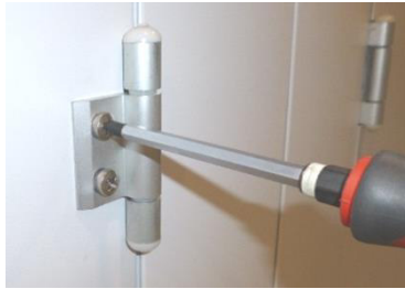
Figure 128: Adjustment of the door panel (EU.T)
