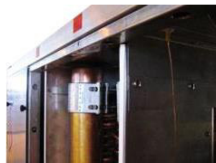
Figure 179: Mounted STRAUB coupling
