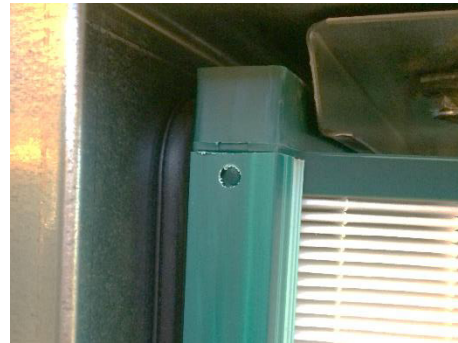
Figure 160: Check, if filter lie on the sealing
