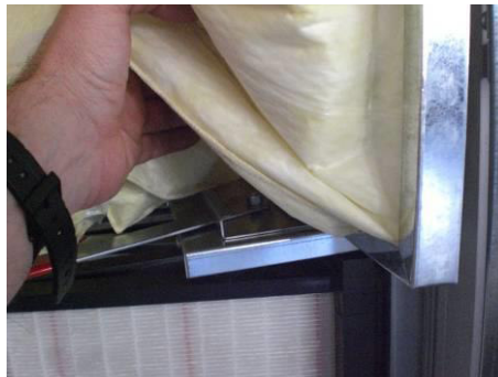
Figure 155: Lifting the filter bags
