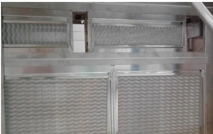
Figure 168: Mounting electrostatic filter
