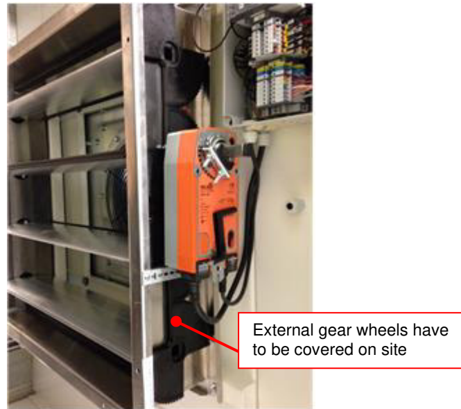
Figure 171: Damper with external gear wheels
