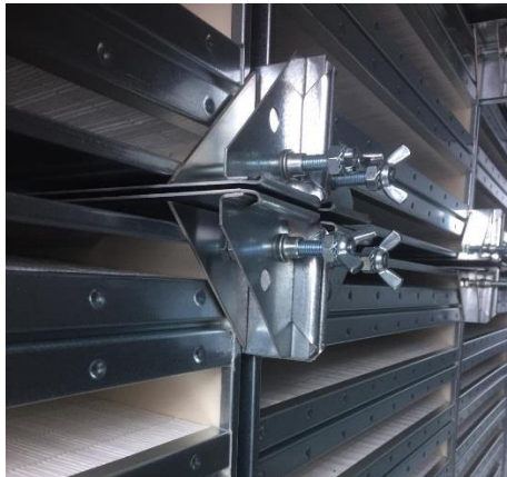
Figure 165: Filter tensioner with pressure plate
