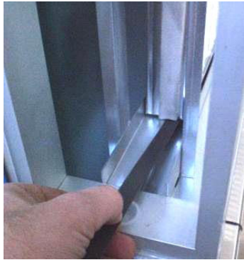
Figure 147: Pulling out the filters
