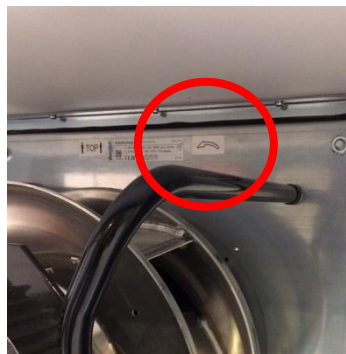
Figure 208: Rotation marking of EC fans
