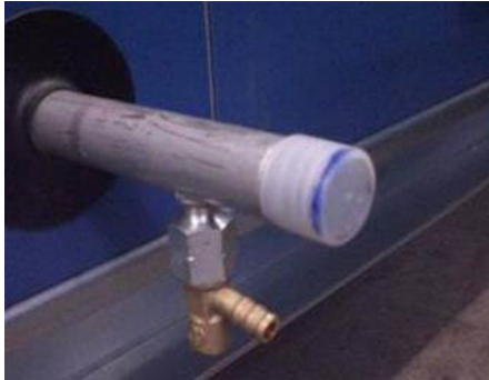
Figure 183: Drain valve
