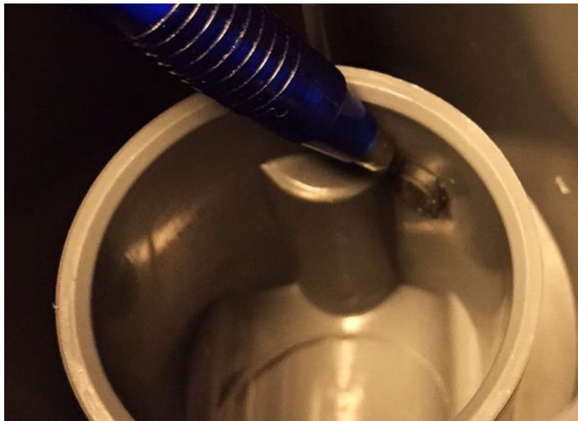
Figure 198: Pressure side installation: remove the black closing plug
