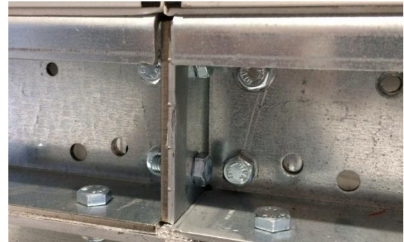
Figure 64: Bolt connection of base frames
