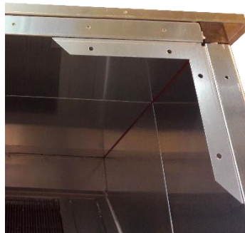
Figure 70: Connection angle
