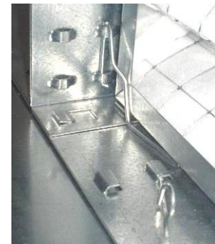
Figure 151: Fixed filter
