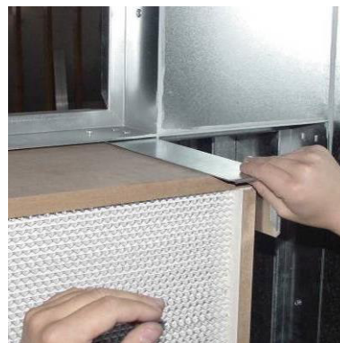
Figur 155: Sett inn filtercellen
