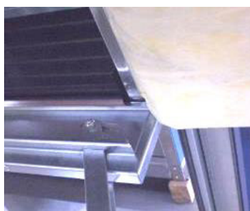
Figur 146: Skyv inn filtrene
