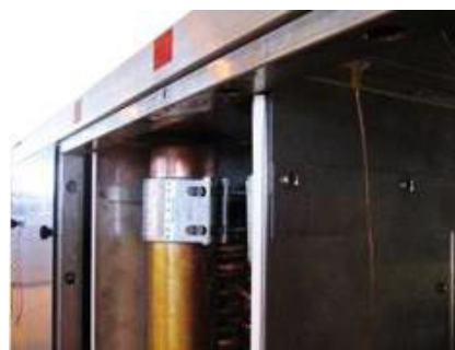
Figur 172: Montert STRAUB-kobling
